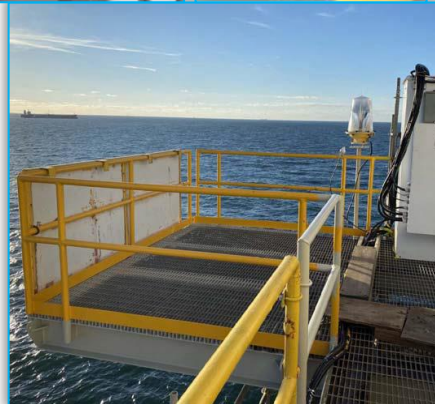
Fabricated and installed additional deck space for FAA equipment
