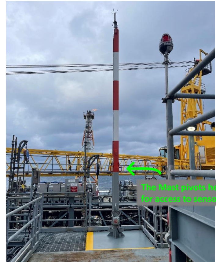
Fabricated and installed a rotating AWOS Wind Sensor Mast
