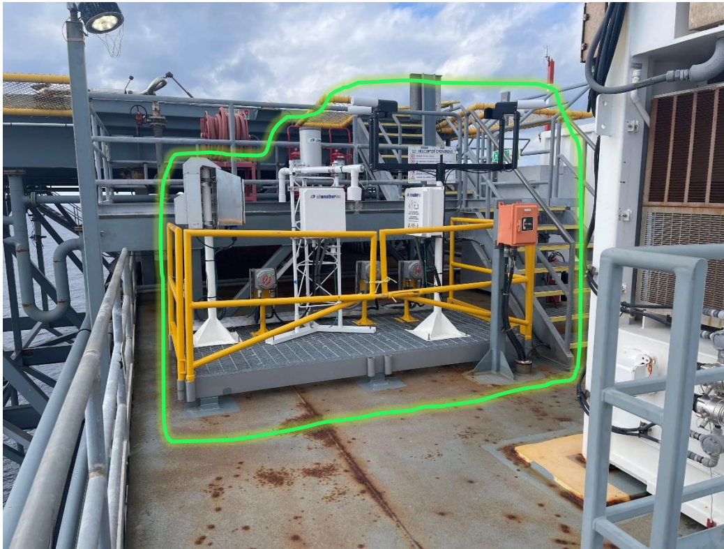
Fabricated and installed AWOS Sensor Suite Skid
